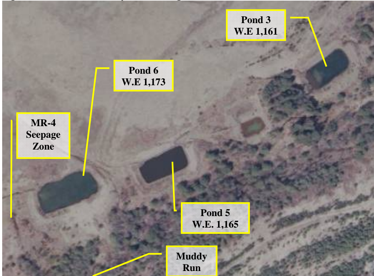
Figure 2. MR-4 Treatment System Existing Conditions
