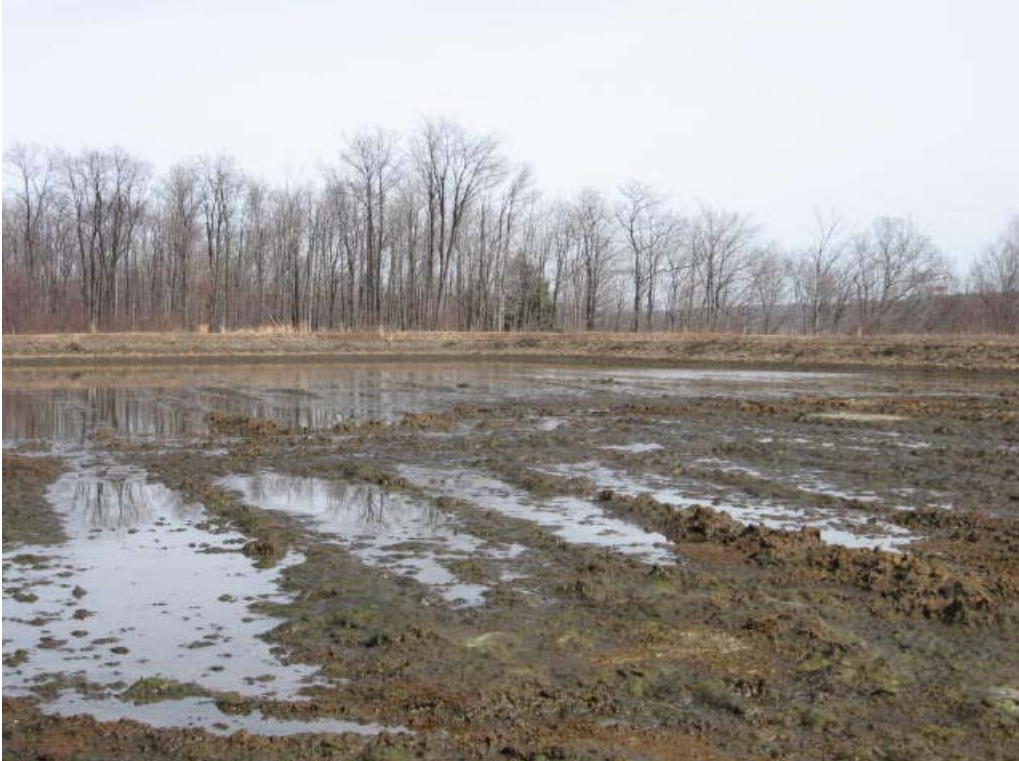
Photo 4. Standing water on top of organic substrate layer in drained Big VFP
